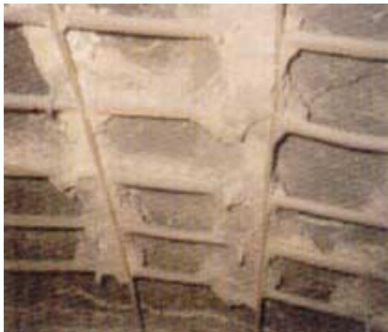
Figure 1: Fire spalling of concrete lining in the Channel Tunnel 1996.<sup>3</sup>
