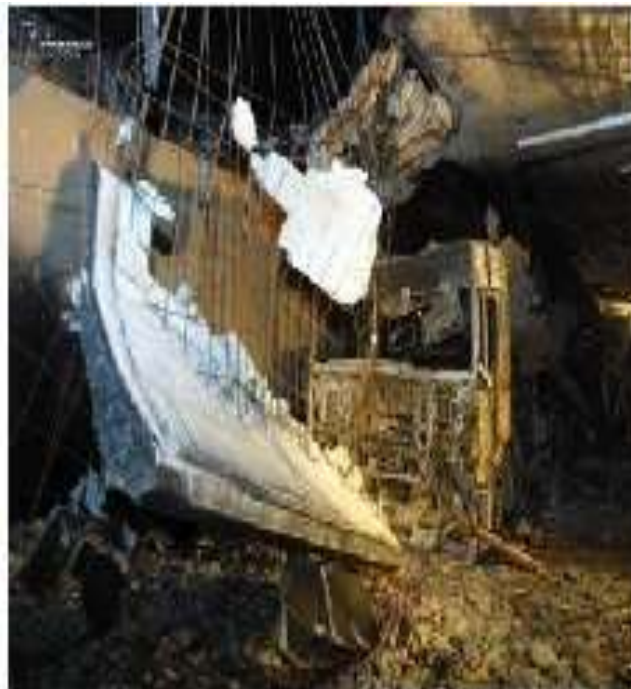
Gotthard Road Tunnel - Switzerland 2001
