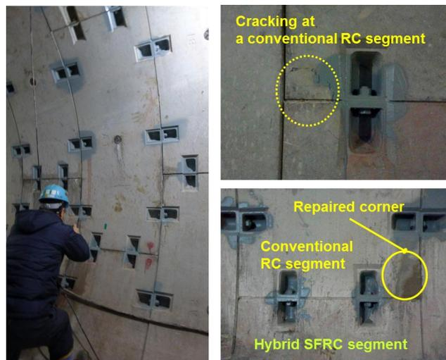
Fig. 11 Hybrid SFRC segment after its field application
