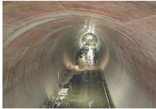
Figure 2: The interior of the North Down's Tunnel, which is coated in fibre-enhanced concrete.
